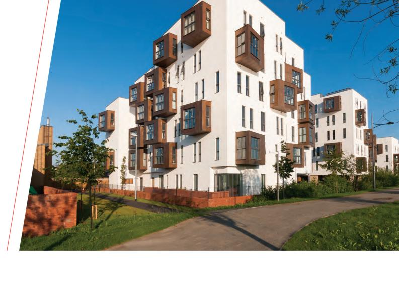
"A big plus for the project was the speed of installation. Each storey typically takes less than two weeks to build and the system works with either steel joisted or concrete floors. Joisted floors result in a lighter structure but concrete floors, such as those used at Mariners Quay, generally provide a higher level of acoustic performance and fire protection."
